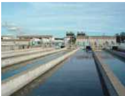
Atlas Copco compressors help supply oxygen to the wastewater-treatment process.
